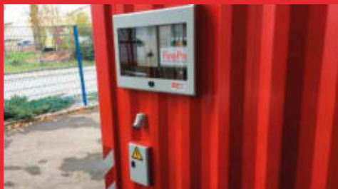
Integrated FirePro fire alarm and Aerosol extinguishing system
